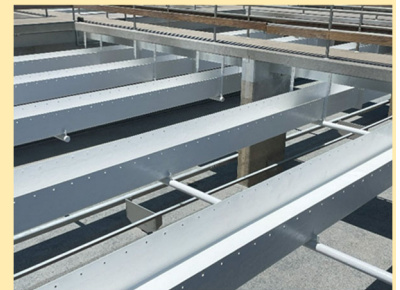
Recoated Steel Launder Mechanisms in Primary Clarifiers
